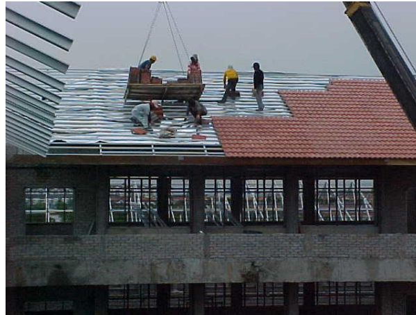
The CORRECT way of installing concrete roof tiles
